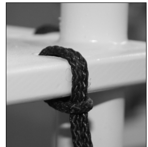
Figure 8 - Kevlar Guy Tie-Down Detail
